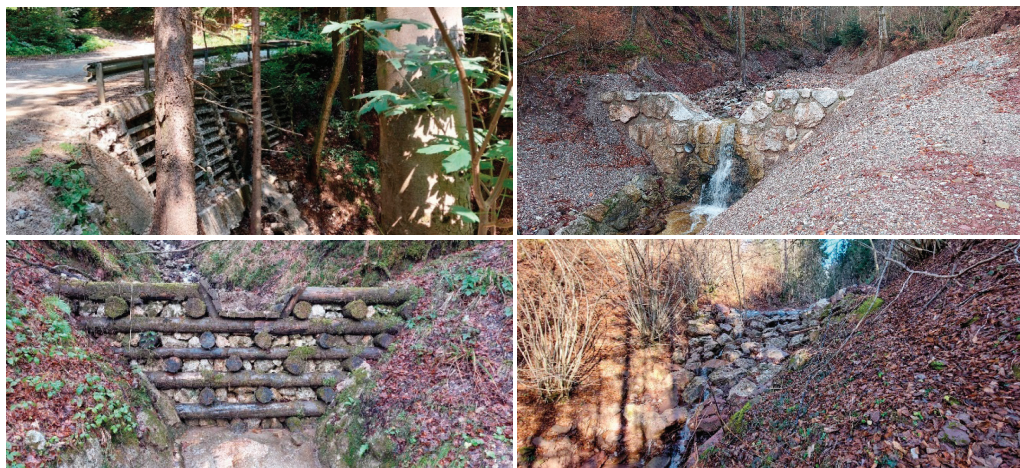
Figure 4: Different barriers serve to mitigate torrential erosion. “Kašta”, a barrier made from wood and rocks, „kašta”, a barrier made from concrete lamellae and rocks, a ramp built with stones, and a weir of stone and concrete structure.
